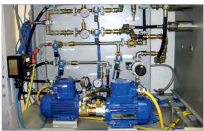
Hydraulic control systems
